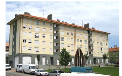
Building "Miribilla" Bilbao
